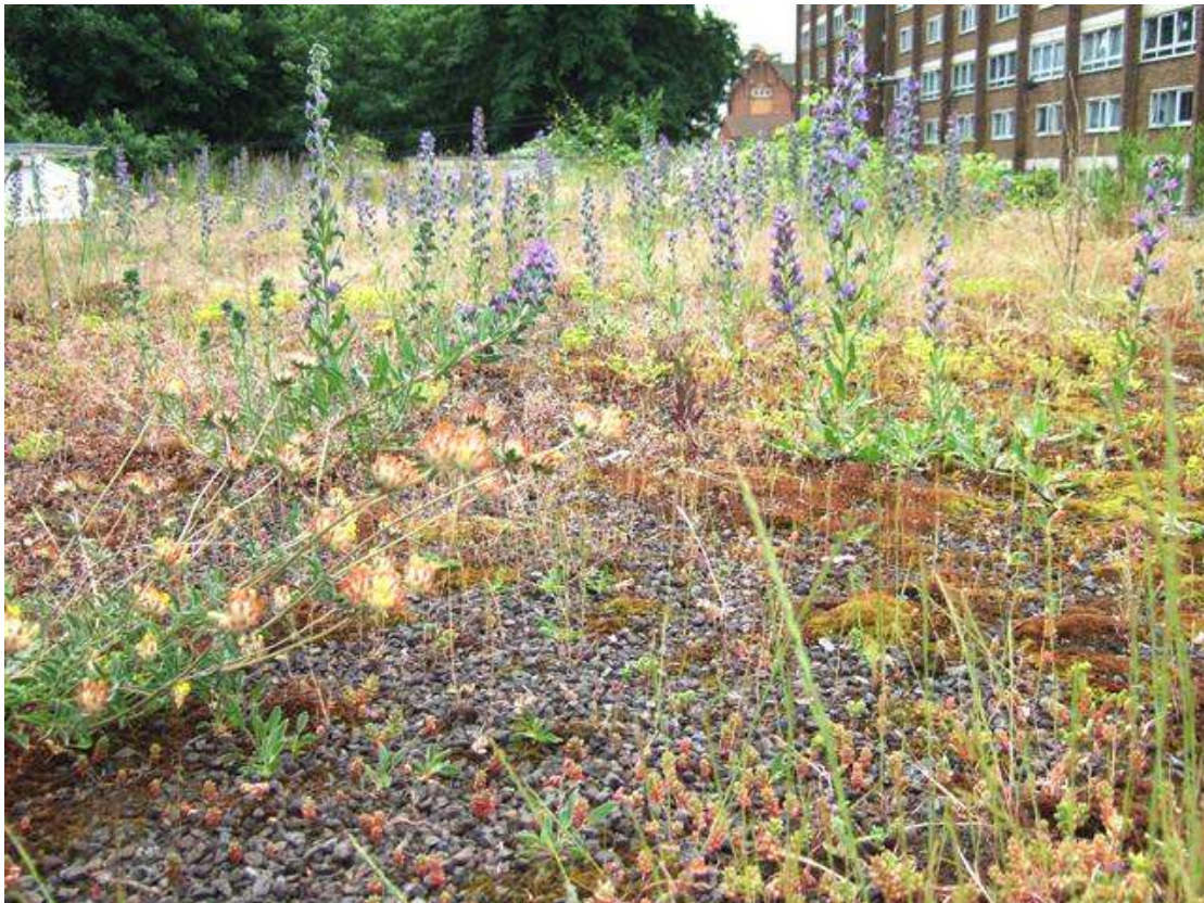
Biodiverse green roof on the Soanes Centre, Tower Hamlets Cemetery Park
